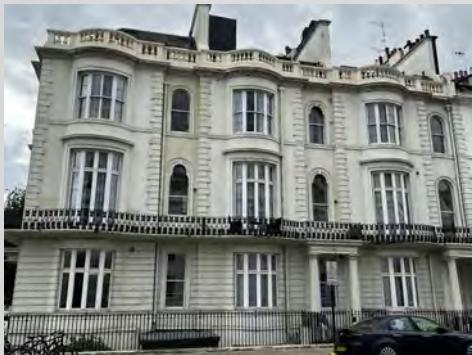
Works included repair and restoration to the masonry and stucco façade, together with full external redecoration of the building. Two stone balconies received specialist strengthening to improve their performance while retaining their original form. As part of these works, sections of the structural steel were replaced and
