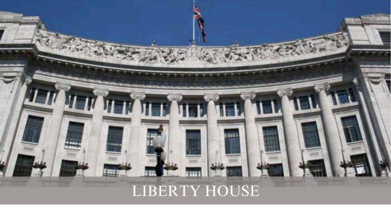
Triton undertook a comprehensive external refurbishment and repair program to the Grade II listed neo-baroque wing at the iconic Liberty department store. Our team used a Decothane Omega 20 system and installed new lead screening to the plant rooms. We replaced the rooflights, renewed the roof and meticulously restored the statuary on the frieze, following a precise specification provided by Adrial Consultancy.
